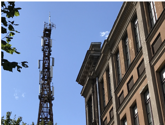
Figure 1: Example base transceiver station (BTS) from with several antennas located close by this Faculty
